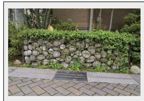
Figure 3 Cage filled with cobble stones with spaces in between
