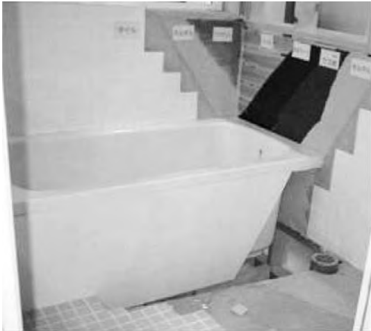
Bathroom built using the conventional construction method
