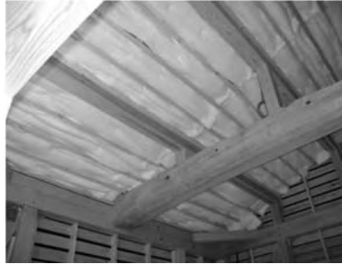
Insulation material on the underside of the roof
