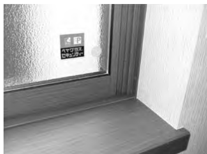
Compound sash of aluminum and resin (laminated glass specification)
