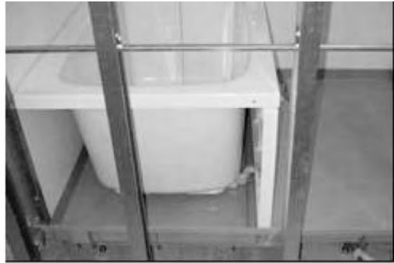
Structural view of a noninsulated type prefabricated bathtub
