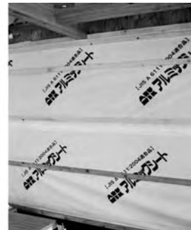
Furring strips for ventilation
