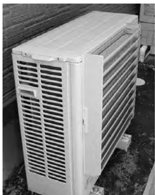
Directional louvers for the water heater
