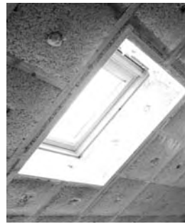
Insulation of roof
