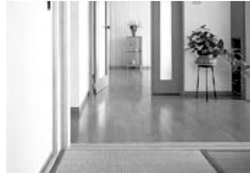
Barrier-free design (flat floor surface)
