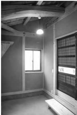
Doma-style (earthen, tiled, or stone-paved) floor and recycled fittings
