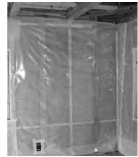
Insulation of exterior walls
